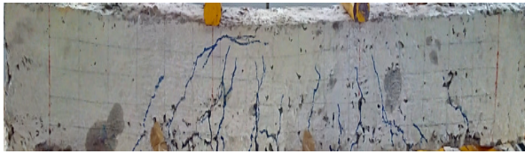
Fig 12 Control beam with after application of load
