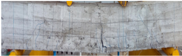
Fig 15 After application of load for lapped beam without gap
