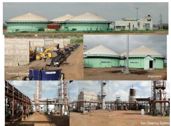
Fig. 2. Biogas / Bio Cng plant
