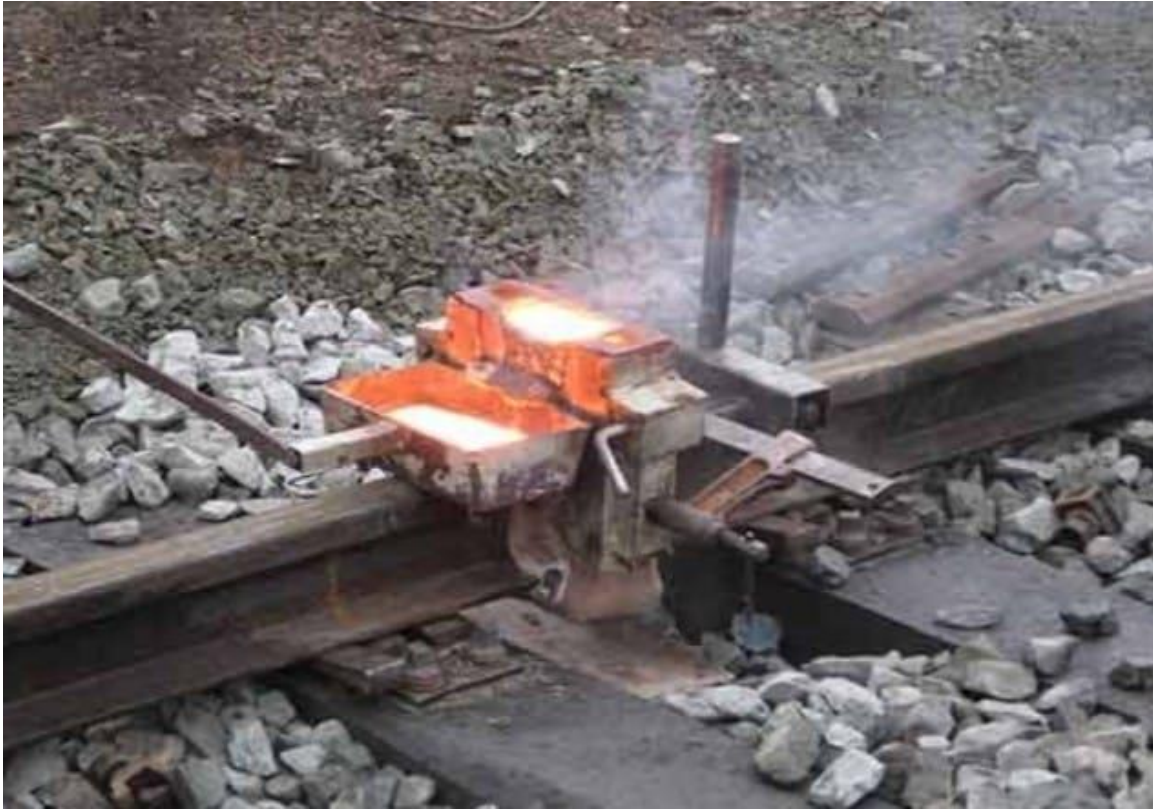
Fig.5: Thermite welding
