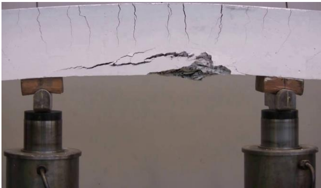
Figure-1 Crack of Beam
