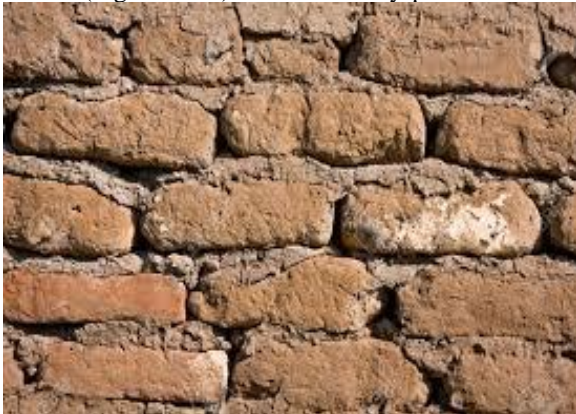
Figure Error! No text of specified style in document.a: Degradation of mud brick walls
